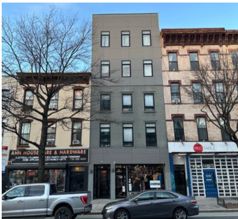
Proponent's condo building, featuring seven dwelling units over one store, outfitted with NFPA 13R sprinklers and served by a single exit, per New York City Building Code 1006.3.2.7 (photo by author)
