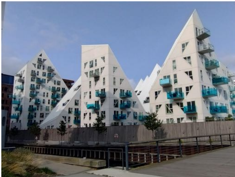
A series of modern, non-combustible single-stair buildings
